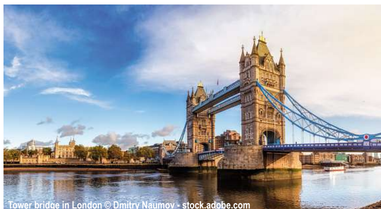
Tower bridge in London © Dmitry Naumov - stock.adobe.com
